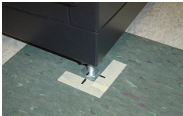
Figure 4-3: Marking Reference Points for a Front Leveler
